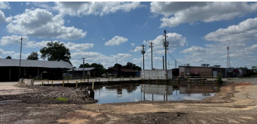
Eight inground docks with dock levelers
